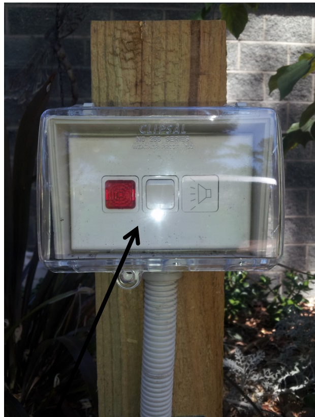
Audio-visual alarm – neon light, buzzer, with a switch to isolate buzzer noise until problem is sorted.
