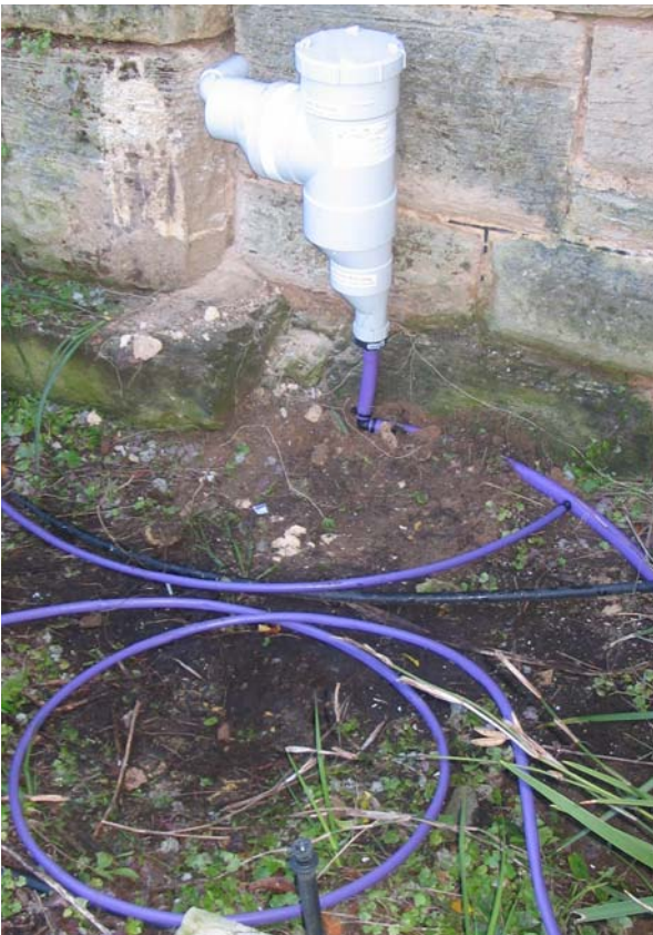
Some photos of typical install – Some dripline can work under gravity but most systems are pumped to gardens.
