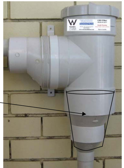
Figure 3. (L) Filter bag inside body. (R) Approximate position of filter bag in body.
